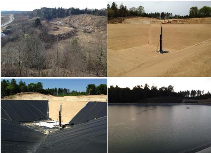
**Fig. 11:** Pictures from implementation of the pit heat storage in Dronninglund (source Dronninglund DH)
