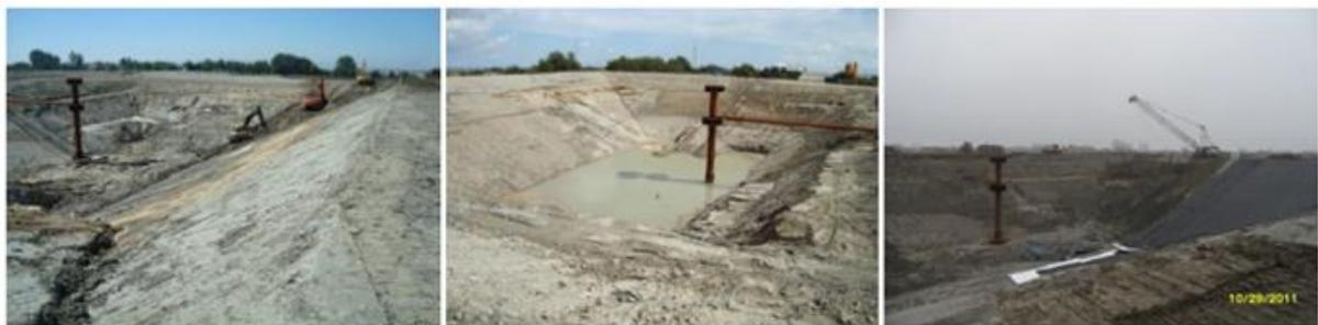
*Fig. 9: Pictures of the excavation process. In the first picture the excavators are preparing the slides for liner implementation. The second picture is a few days after a cloud burst. In the last picture a cable excavator is digging up mud from the bottom while the liner implementation has begun (Source: PlanEnergi)*
